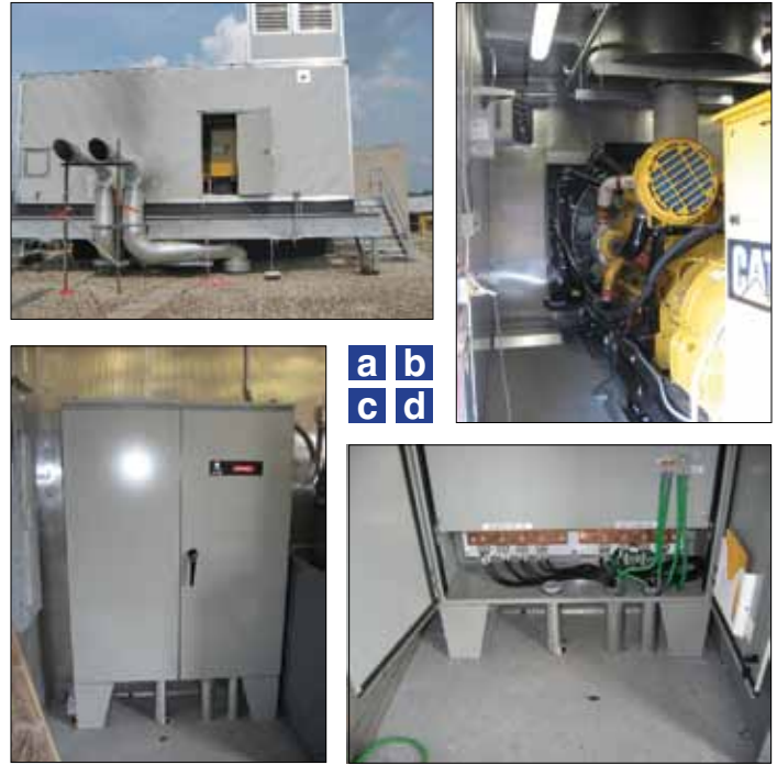
Figure 7a: Magee rooftop installation
